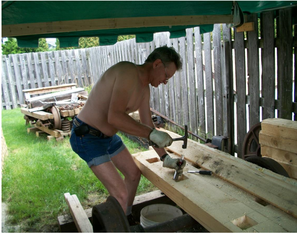
4- Cutting Mortis and Tendent joints on the beams
